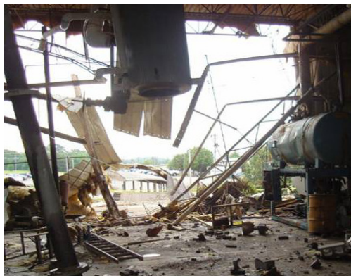
Remote boiler maintenance enables to avoid disasters...
